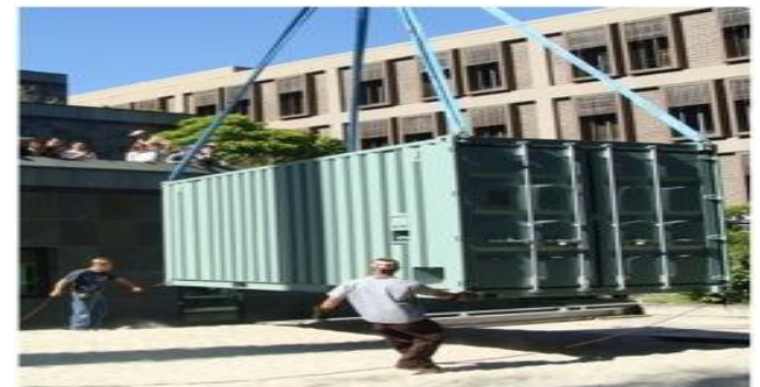
The Million Server Datacenter Providing IaaS
